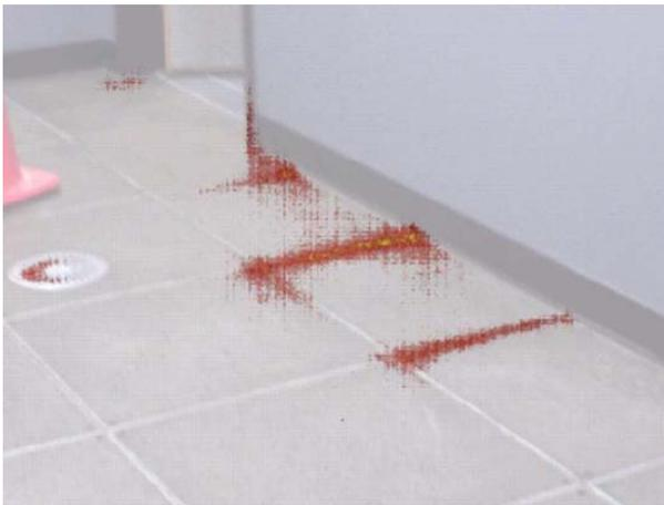
Image 2: Floor to wall joint is leaking and there is separation of some tile joints of the UFAD system
